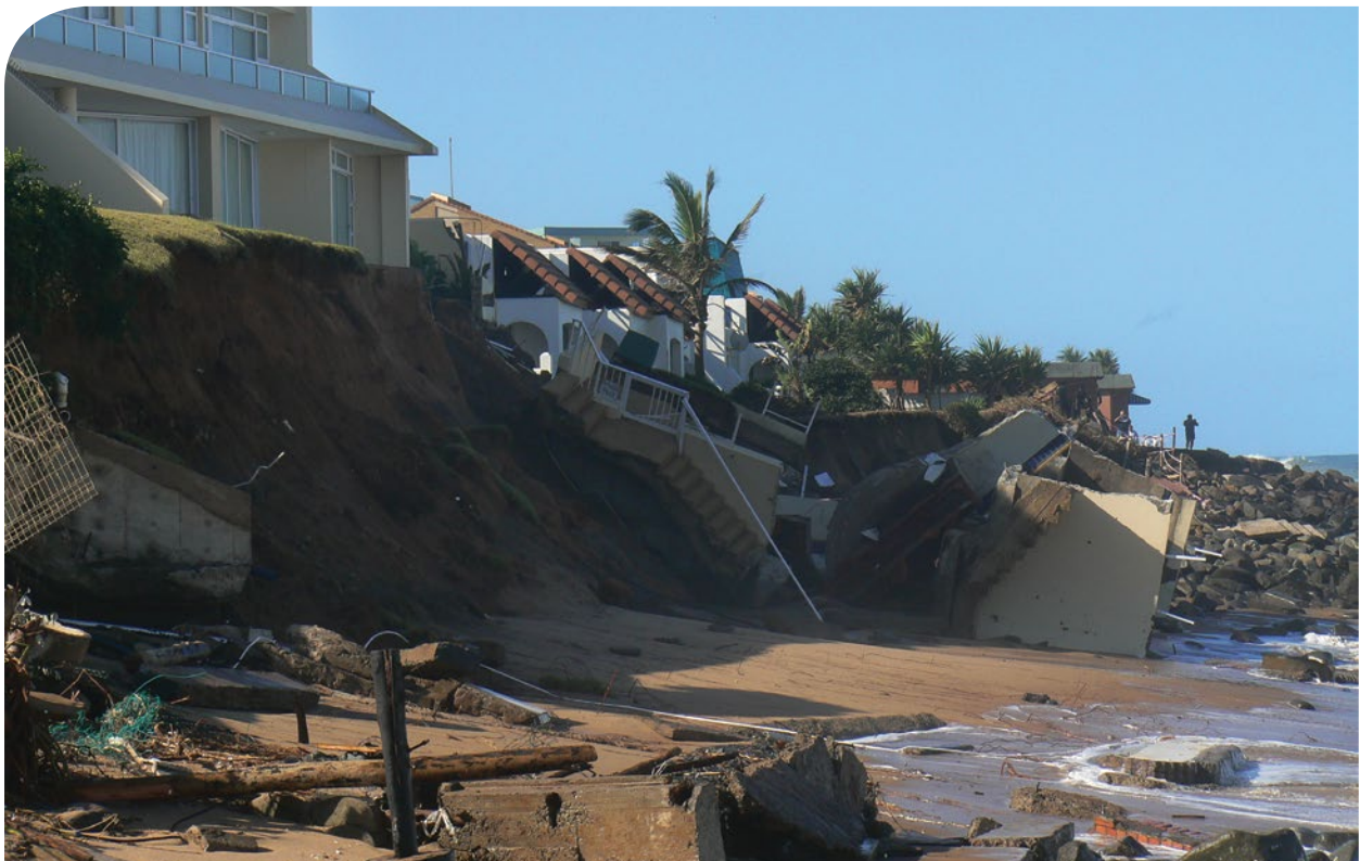
Inappropriate coastal development undermines the resilience of coastal ecosystems and increases the risk of infrastructure failing in the face of natural hazards. © Linda Harris.
