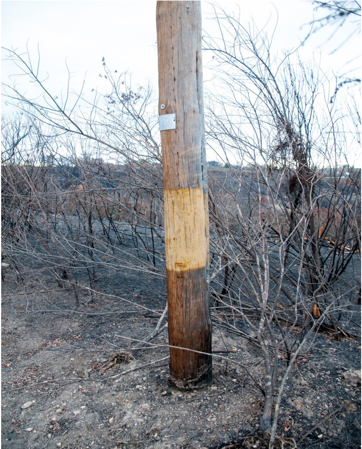
Figure 472: The Western side of pole in Figure 46 showing less severe fire damage
