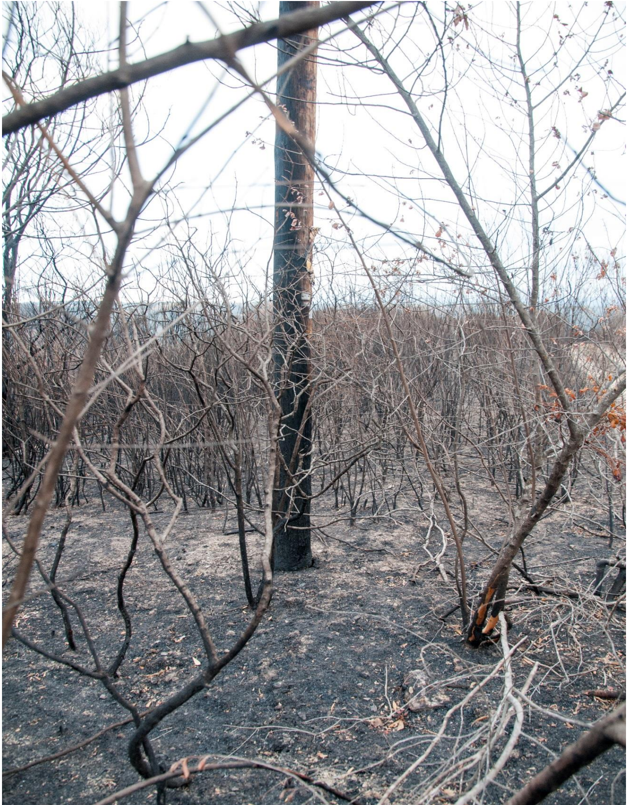
Figure 43: An electricity pole. Note the fire damage on the Eastern side
