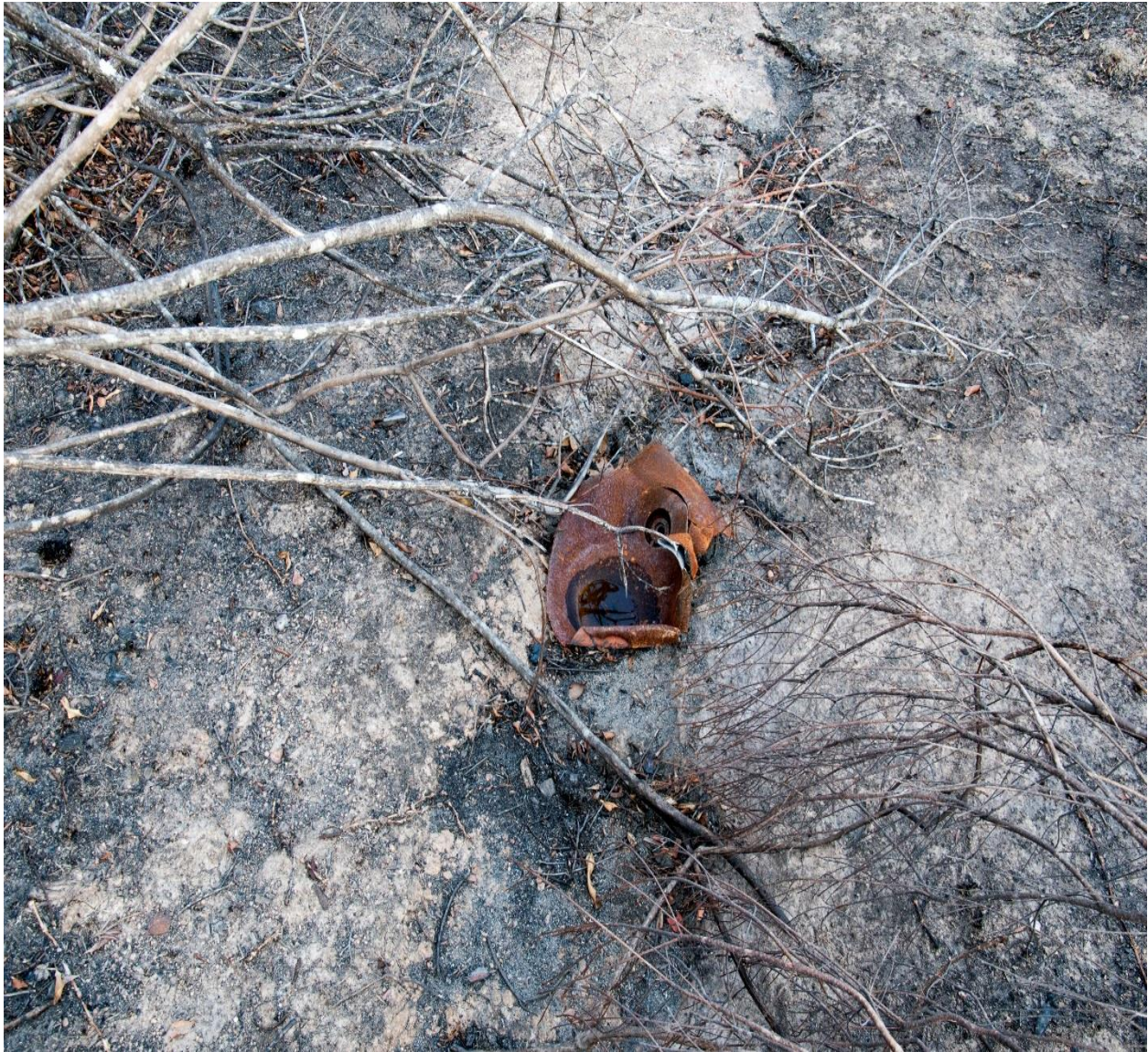
Figure 56: Remains of a LP Gas cylinder found in the access path
