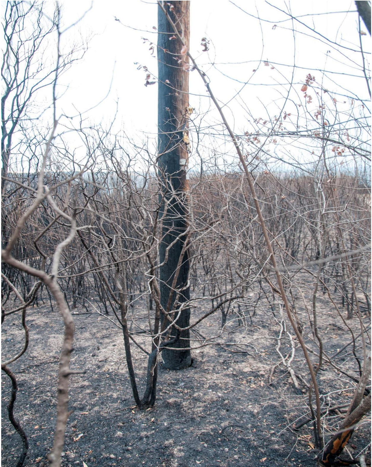
Figure 44: An electricity pole. Note the fire damage on the Eastern side
