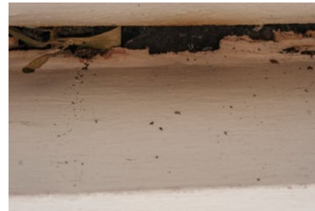
Above: This image shows how the smallest vulnerability can lead to a home burning down. This photo shows what's left of a burning leaf which had collected over time with other organic materials. Embers blowing into this area, between the gutter and fascia board, caused the leaves to ignite which caused the fascia board to begin burning. Fortunately the homeowner noticed this and extinguished it before the fire could cause serious damage. This small vulnerability could have resulted in the home being lost.
