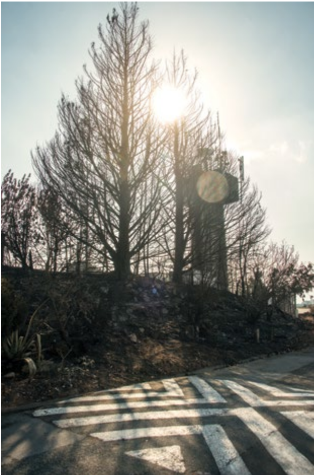
Above: Communication infrastructure in the WUI area of Knysna Heights.
