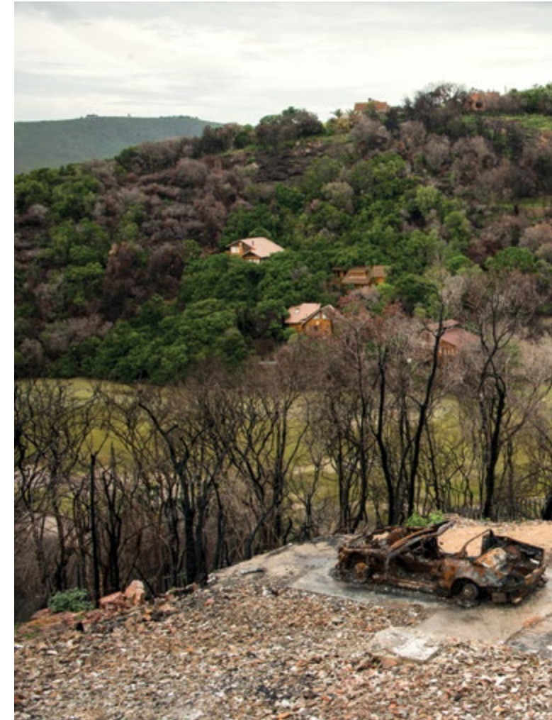
The positioning of a home on a slope can have a dramatic impact on whether a home will be resilient to the possible damage of radiant heat and ember attack during a wildfire. Many homes in Knysna were built in incredibly vulnerable positions with little or no regard for risk reduction measures.
