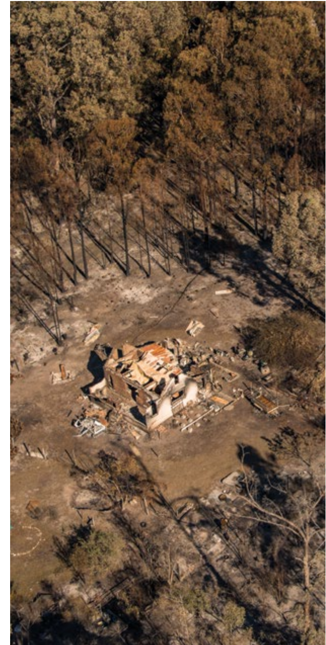
Right: A home in Belvidere situated in the middle of tall gum trees lies in ruins. Despite there being a cleared area around this home, there is the possibility that large embers flew off the trees and found a vulnerable access point into part of the home, leading to its ignition.
