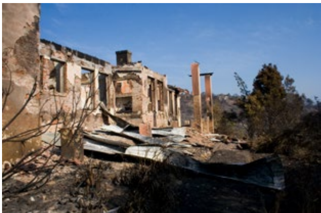
Above: This home was positioned on top of a slope and had large and dense vegetation in close proximity. Heat and flames rushing up the slope would have had a direct impact.
