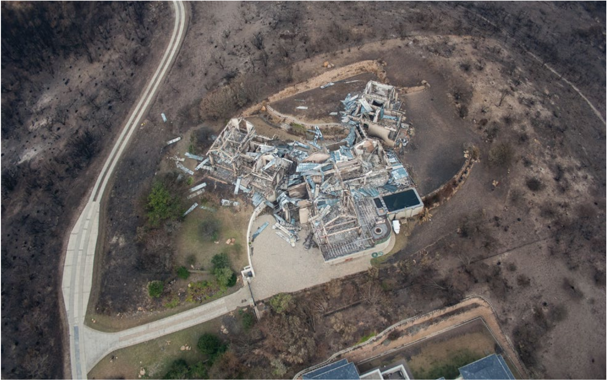
Above: A large home in Pezula Estate, outside of Knysna reduced to rubble. It is likely that the position of this home, on a slope with the close proximity of the vegetation contributed to its destruction.
