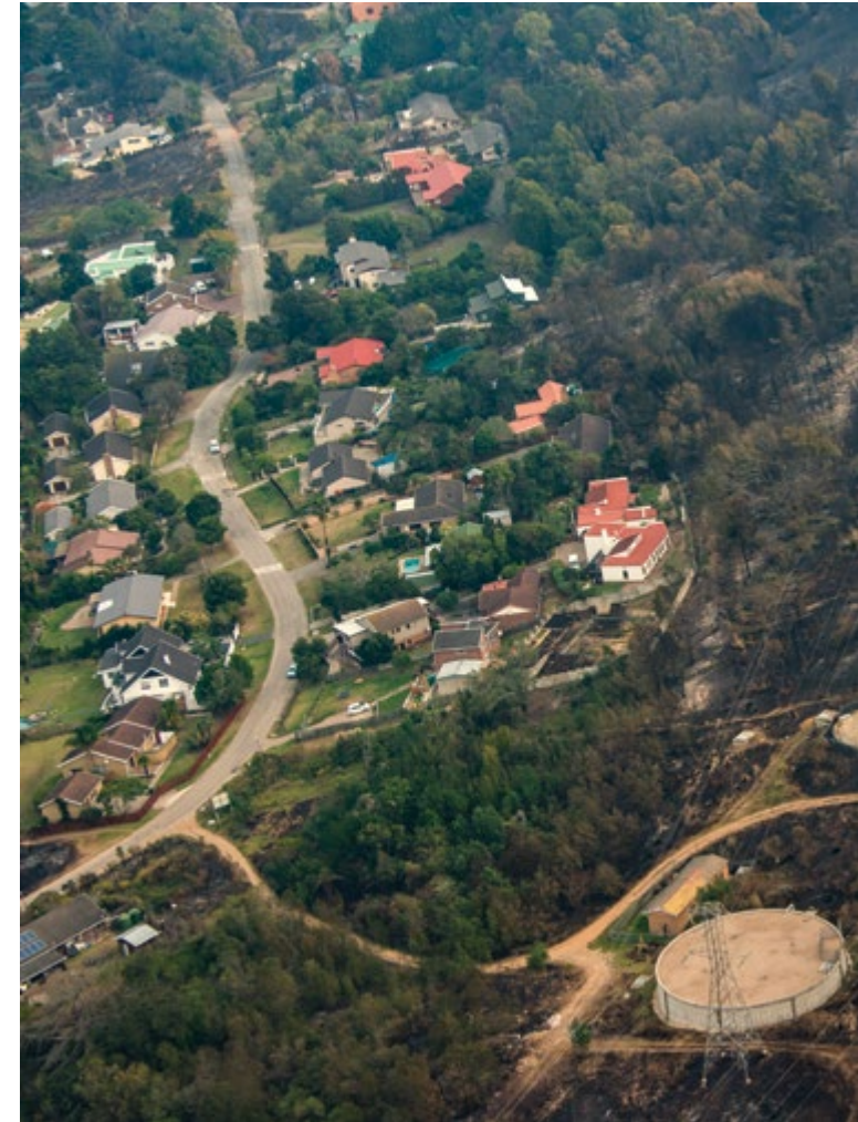
Above: Homes and vital town infrastructure are both found within the WUI. Here you can see how the Knysna Fires has burned in an area near power lines, water reservoirs and homes. A holistic risk reduction strategy for all assets and infrastructure is required.
