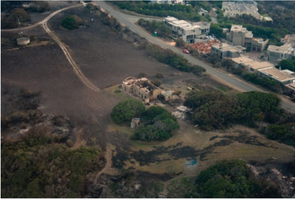
Above: The Robberg home in the centre of the image above was destroyed by direct flame contact but the homes on the other side of the road (acting as a barrier) did not suffer any damage.
