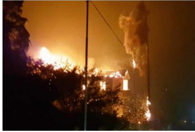
Above: The images above (taken from a video) show a palm tree nearby the Knysna Town that has ignited from embers. This palm tree ignition has subsequently compromised the building next to it as the embers from the palm tree caused the structure to ignite. Photo Source: Jacky Stassen, Knysna Fire Stories book (2017)
