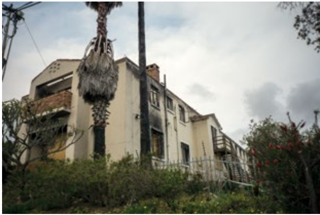
Above: In comparison these images were taken during a visit to Knysna by Vulcan Wildfire Management in November 2017. There was no evidence of a burn scar in the neighbourhood surrounding the destroyed structure and further analysis proved that it was embers which caused the palm tree and then the structure to ignite.
