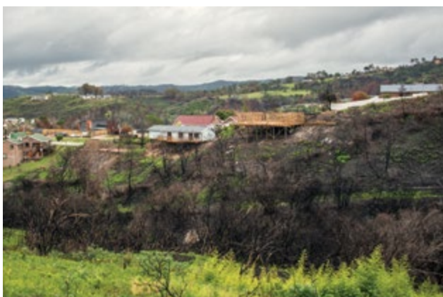
Above: Homes in the Knysna area being rebuilt seemingly with no regard to future wildfire risks. They are being constructed out of the same easily flammable materials and are placed in a dangerous position on a slope with decking extending out over the slope. Without the creation of Defendable Space and once the vegetation grows back, the flames and embers from a fire moving up the slope and the valley could easily reach under the deck causing it to ignite. While a rebuild is important it is equally important that lessons are learned and wildfire risks are understood.
