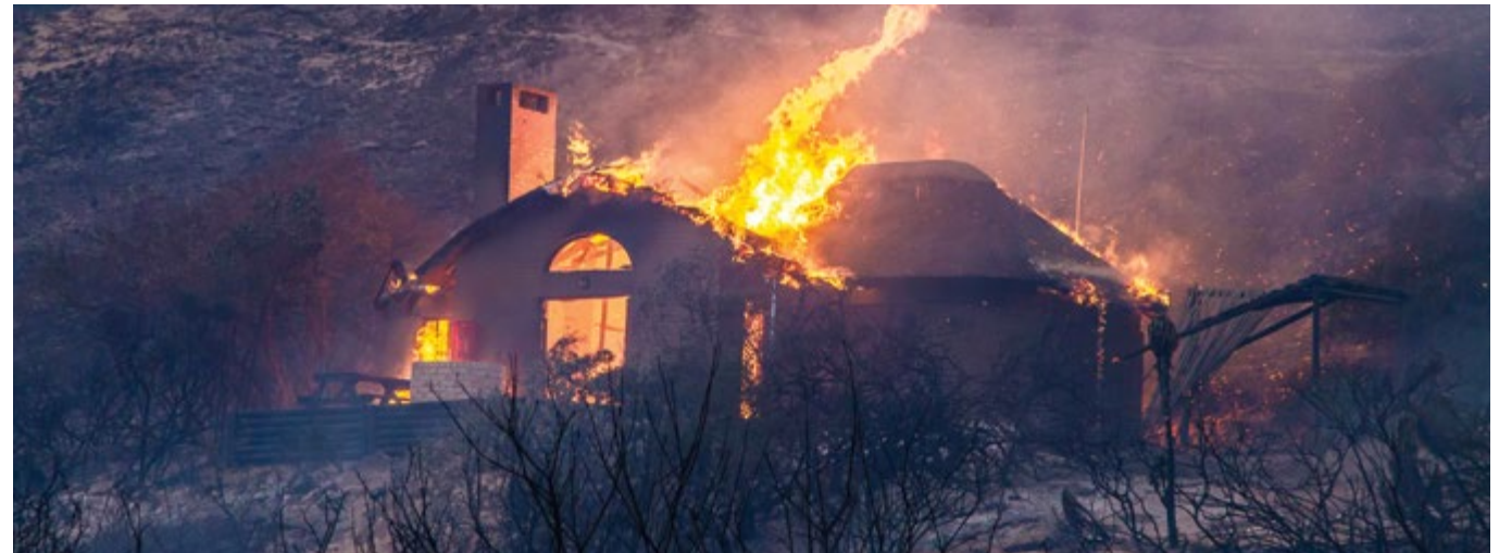
Above: Shows the neighbouring home (to the two wooden homes destroyed in the image left). With extensive heat damage to the outer wall (closest to the neighbouring wooden homes) this suggests that this home was destroyed by structure-to-structure ignition. The extreme heat from the homes burning, as well as the strong prevailing wind direction promoting transfer of heat meant this home stood little chance.
