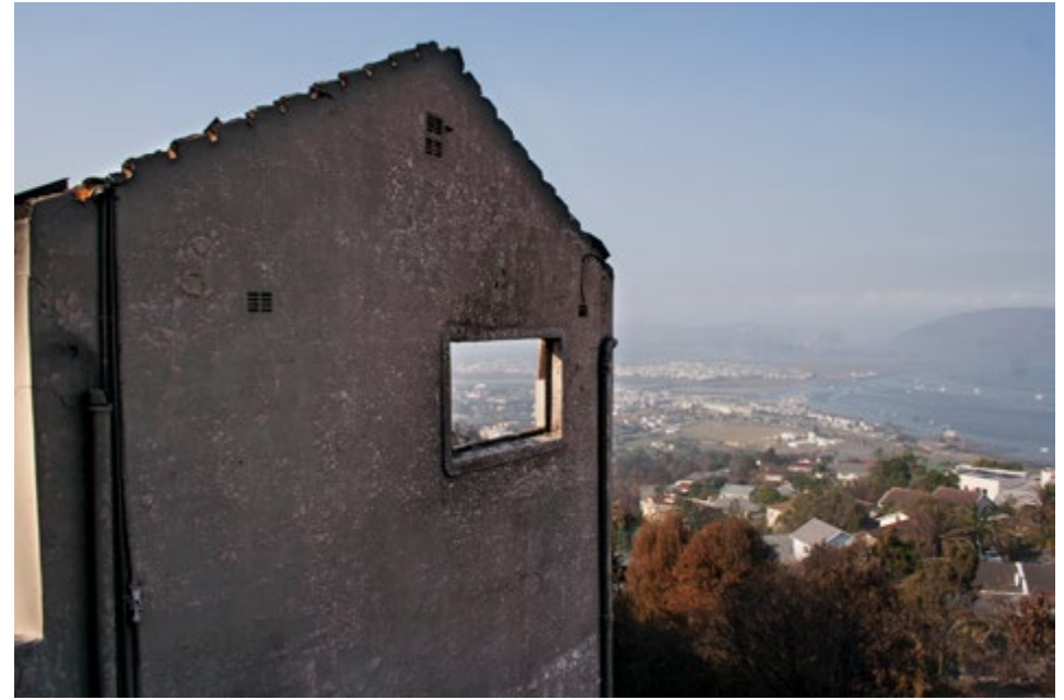
Above: Shows the neighbouring home (to the two wooden homes destroyed in the image left). With extensive heat damage to the outer wall (closest to the neighbouring wooden homes) this suggests that this home was destroyed by structure-to-structure ignition. The extreme heat from the homes burning, as well as the strong prevailing wind direction promoting transfer of heat meant this home stood little chance.
